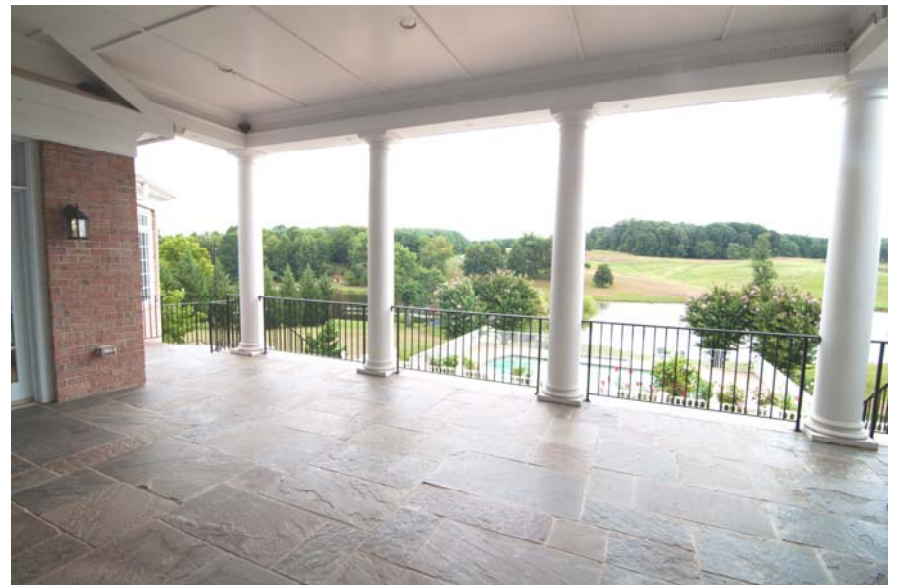
Rear Veranda with Slate flooring
